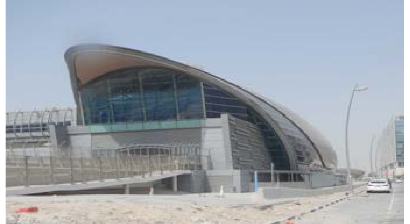
UAE Exchange station prior construction of new entrance
