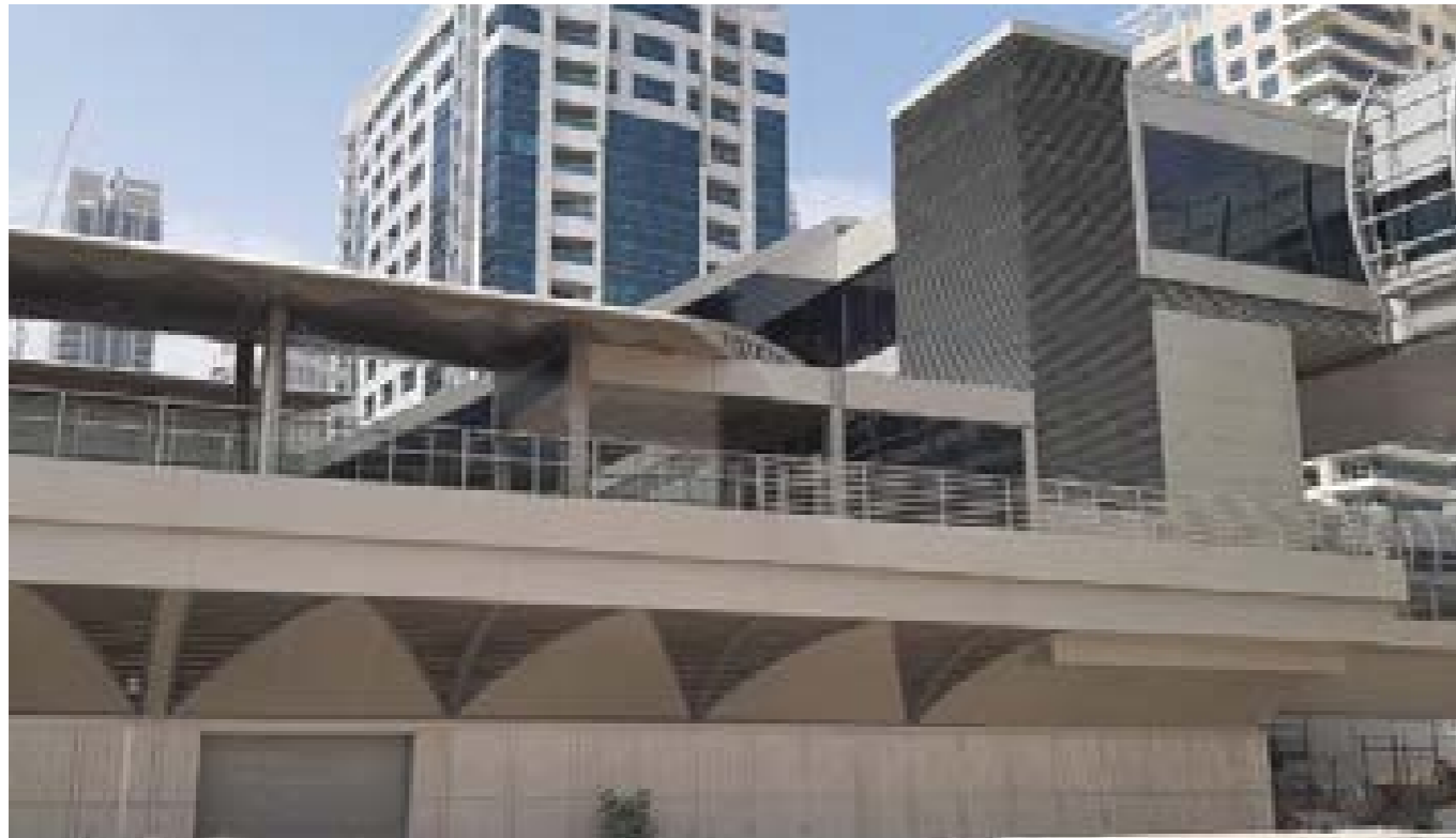
Old connection (lift) between Metro footbridge and tram station
